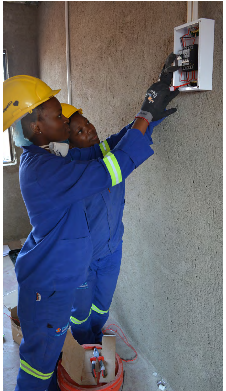
SKILLS TRANSFER: Ms Dimakatso Ngwane and Ms Tercia Mngwenya testing the meter box immediately after installation.
